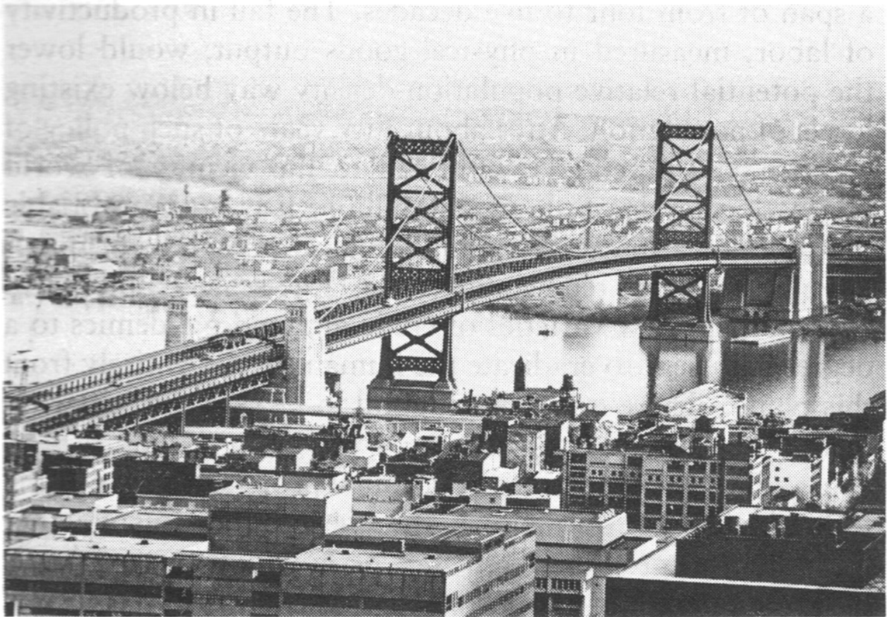
It can be demonstrated that progress is a necessity. Above: Ben Franklin bridge between Camden, New Jersey, and Philadelphia.
